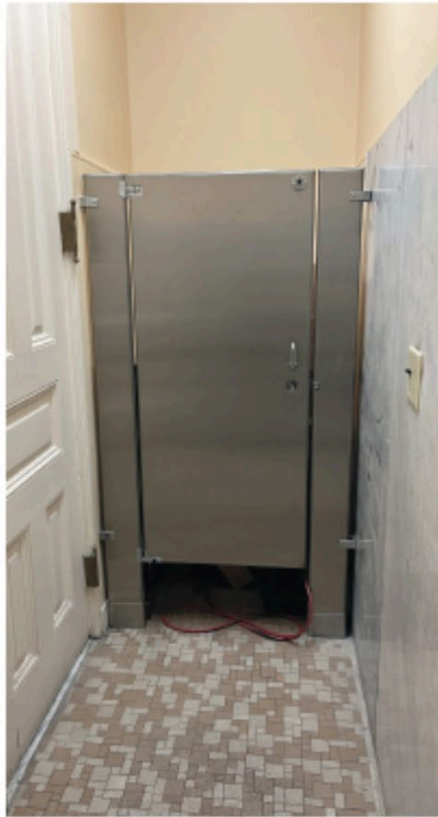
Many of the public toilet rooms in the Capitol have been added over time in awkward locations. These toilets do not provide a visitor experience consistent with the historic spaces of the Capitol.
