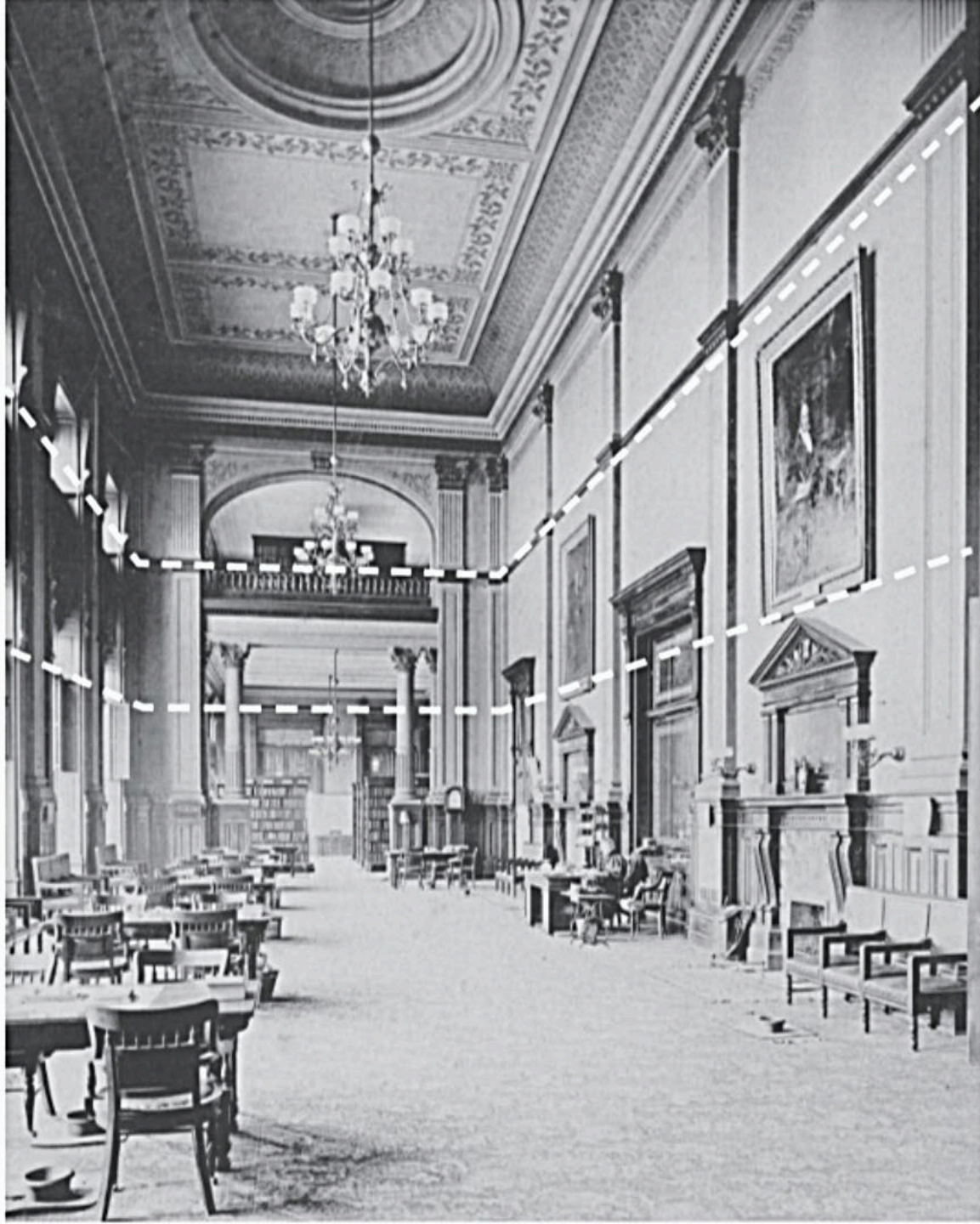
Historic photograph of the Capitol Library. It has since been obscured by the construction of infill floors and mezzanines - shown via the white dashed lines overlaid. Image courtesy of the Atlanta History Center.
