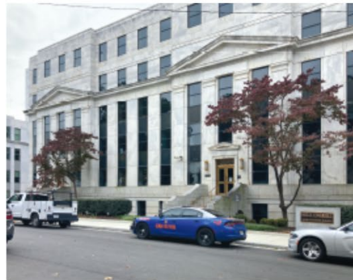
Site for Project Option 1 - the existing Coverdell Legislative Office Building (CLOB)
